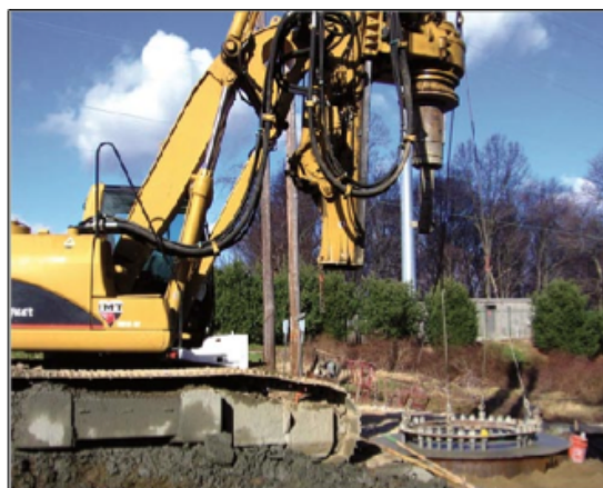
Structure Foundation Installation
