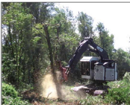
Transmission Corridor Clearing
